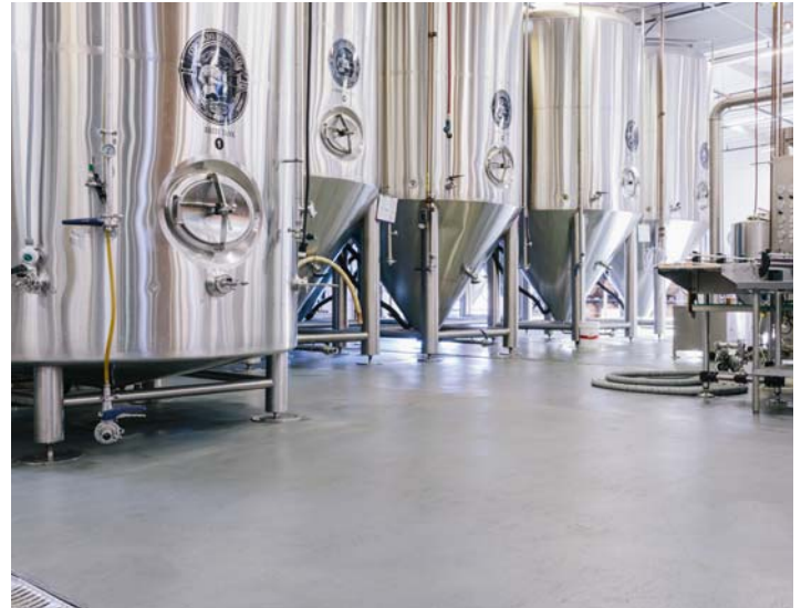
Stonclad UT, a textured polyurethane mortar floor stands up to thermal shock and thermal cycling.
